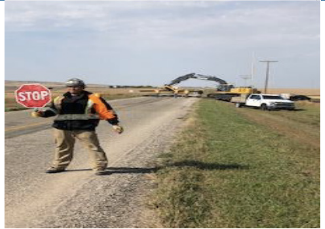
Flaggers were used to move equipment – SF 126 – Sept 7, 2018
