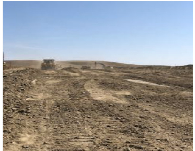
Grading in Heritage Area – km 222+300 – Sept 6, 2018
