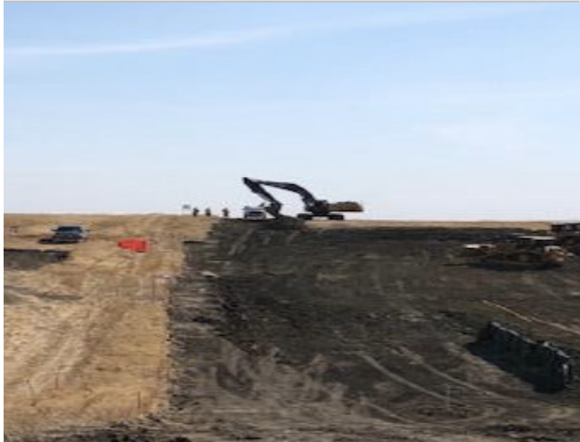
Excavator stripping soil – km 236+800 – Sept 6, 2018
