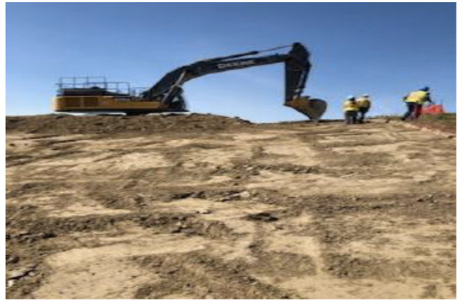
Topsoil being stripped – km 222+648 – Sept 5, 2018
