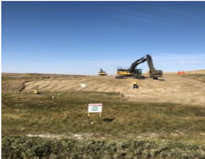
Seconds being stripped - km 222+650 – Sept 6, 2018
