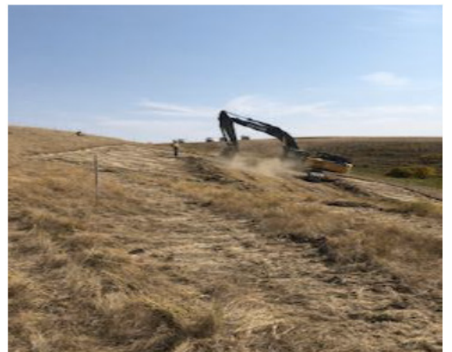
Stripping topsoil – km 222+800 – Sept 7, 2018
