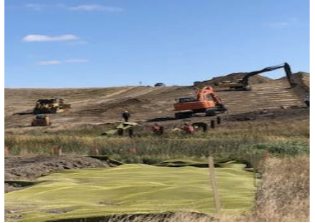
Crew laying geo tec – km 255+100 – Sept 5, 2018
