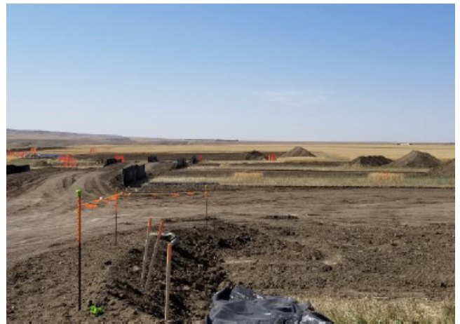
Ramps are built - km 223+675 – Sept 6, 2018
