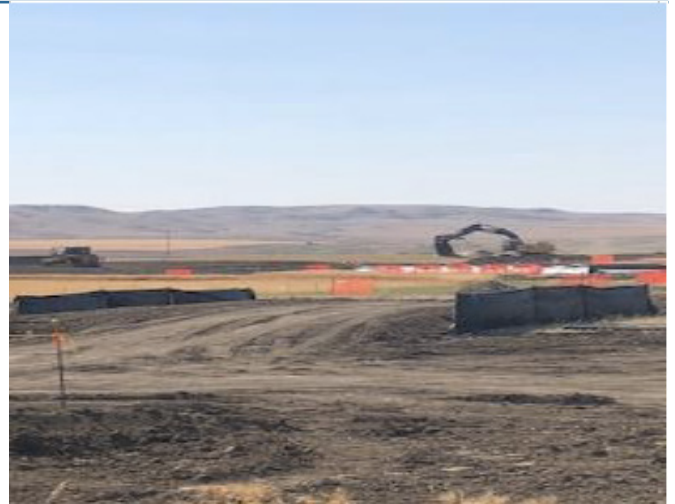
Excavators working on ROW – km 236+478 – Sept 6, 2018
