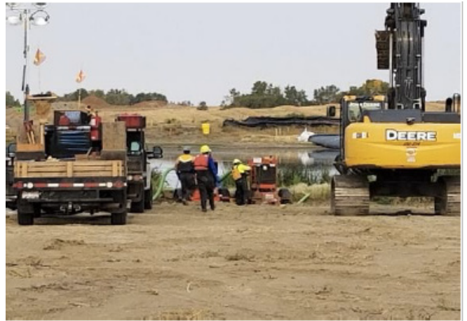
Building Aqua dam - km 165+300 – Sept 8, 2018
