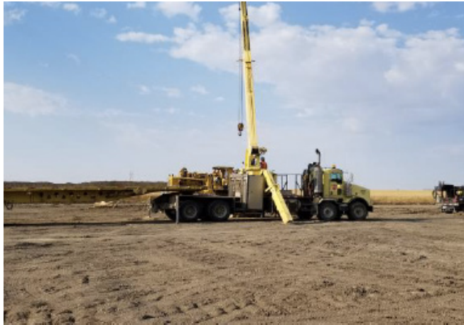
Breaking down boom – km 183+420 – Sept 7, 2018
