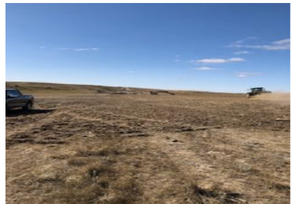
ROW tilled and stripped – Km 222+580 – Sept 4, 2018
