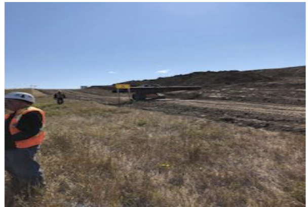
Bobcat stringing out screw piles – km 255+000 –Sept 4, 2018
