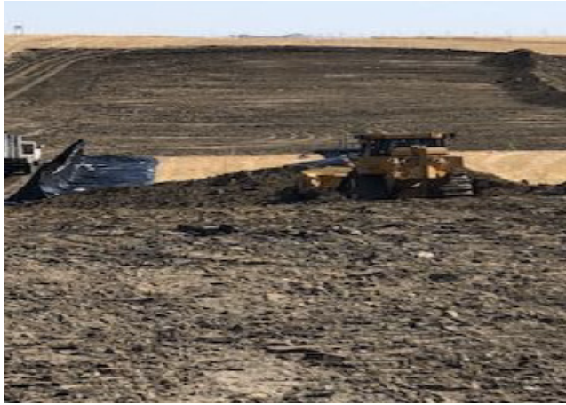
Dozer building access ramp for drainage – km 236+700 – Sept 5, 2018
