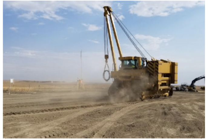
Equipment crossing - km 193+775 – Sept 7, 2018
