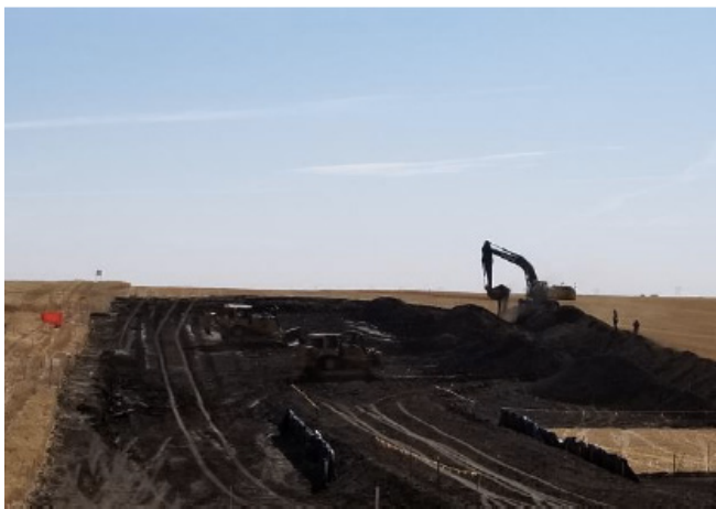
Equipment moving dirt - km 236+650 – Sept 6, 2018
