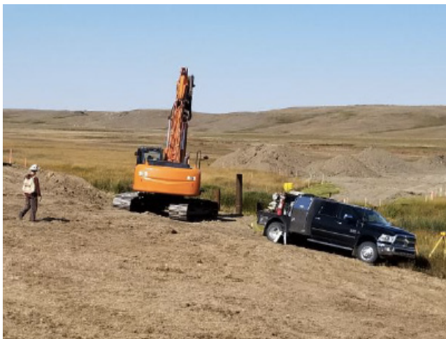
Installing screw piles - km 255+175 – Sept 5, 2018
