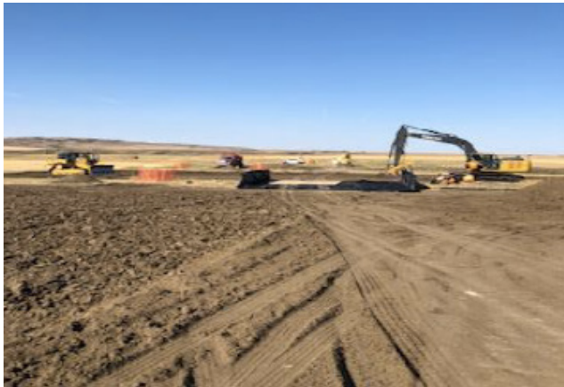
SaskTel Ramp being constructed – Sep 5, 2018
