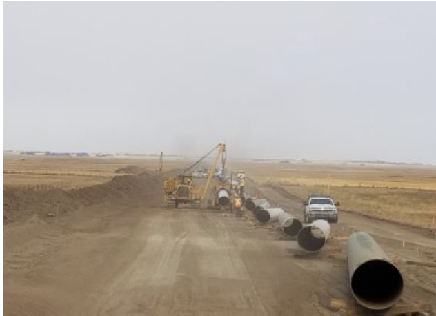
Bending Crew - km 158+270 – Sept 8, 2018
