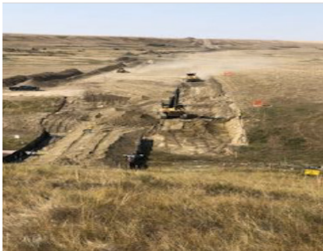
Access ramp and crew grading ROW on Sept 7, 2018
