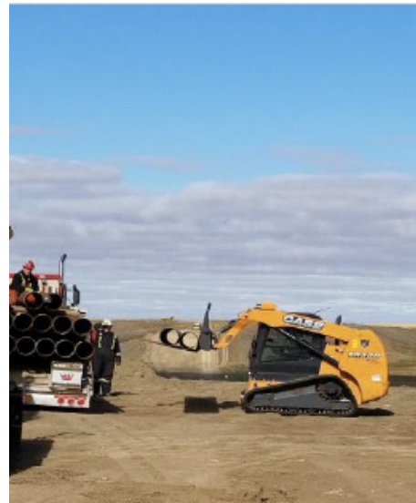
Offloading screw piles – km 255+ 350 – Sept 4, 2018
