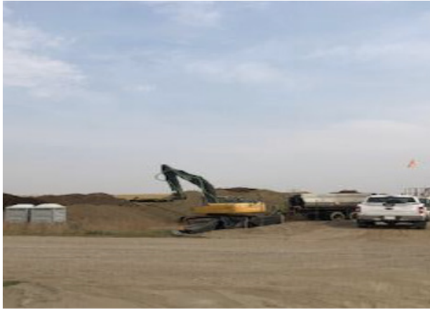
Excavator filling tank – SF 102 – Sept 8, 2018
