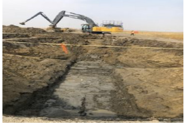
Excavator digging bore bay – km 176+364 – Sept 8, 2018
