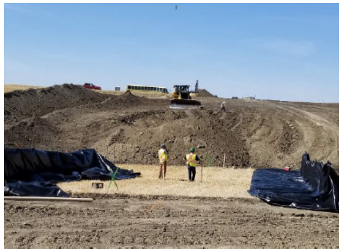
Ramp installation – km 236+740 – Sept 5, 2018
